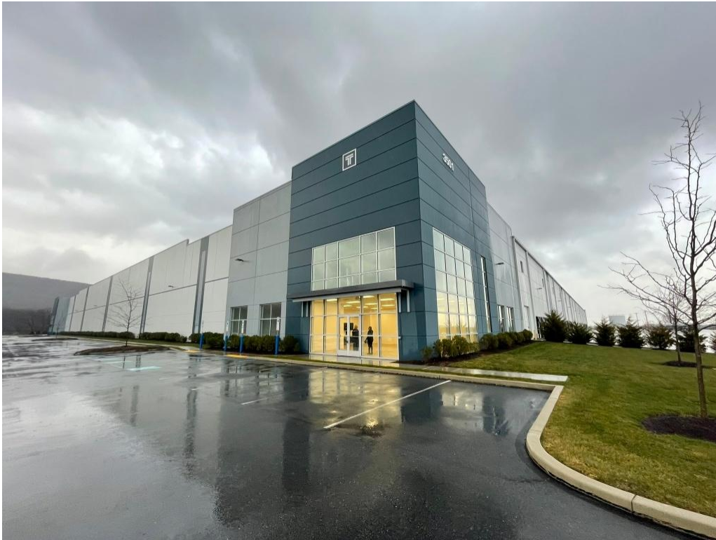
Figure 6. South and west sides of the building at main entry point.
