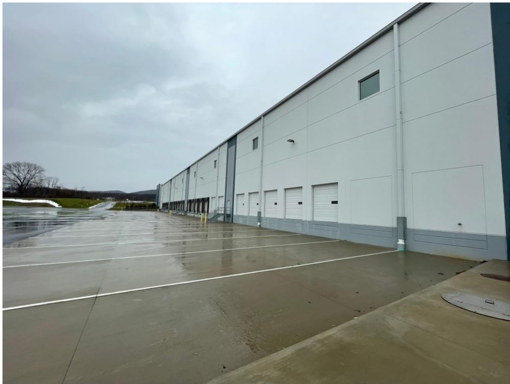
Figure 7. South side of building.
