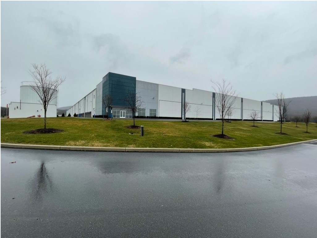
Figure 8. South and east sides of building.
