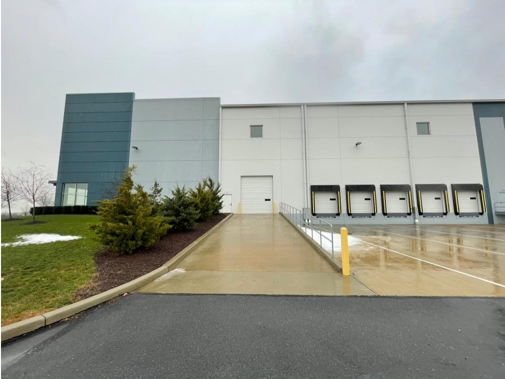
Figure 9. North side of building.
