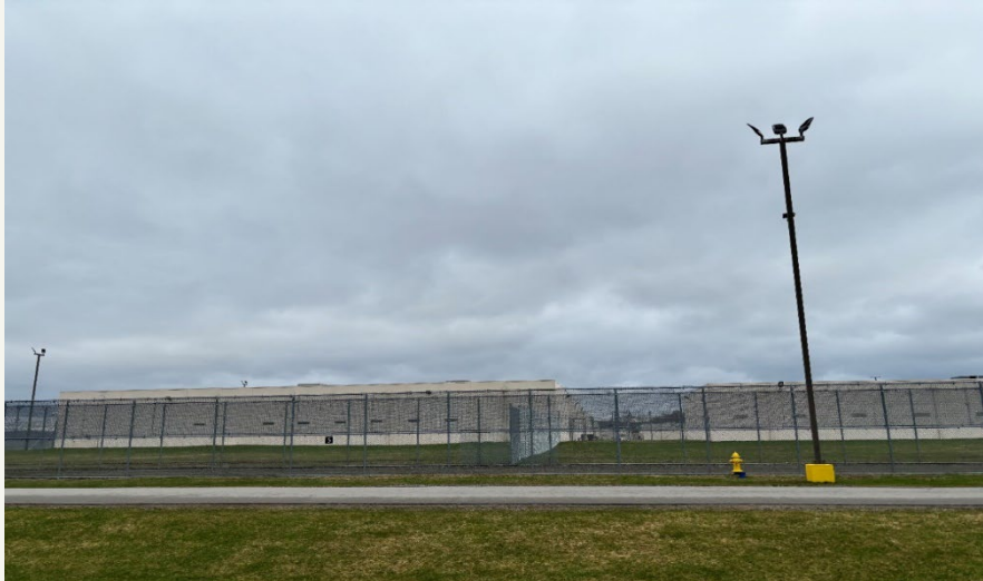
Moshannon's no-climb fence upgraded for ICE
